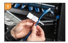
Place adhesive side of label against wire with only the tail touching the wire.
