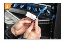
Fold tail over the wire and attach to the exposed adhesive of the bottom label panel.
