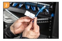
Fold tail over the wire and attach to the exposed adhesive of the bottom label panel.
