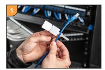
Place adhesive side of label against wire with only the tail touching the wire.
